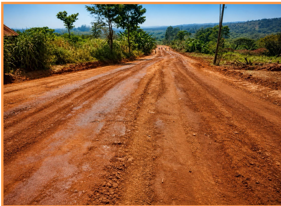
One of two new Tulu Kapi access roads
